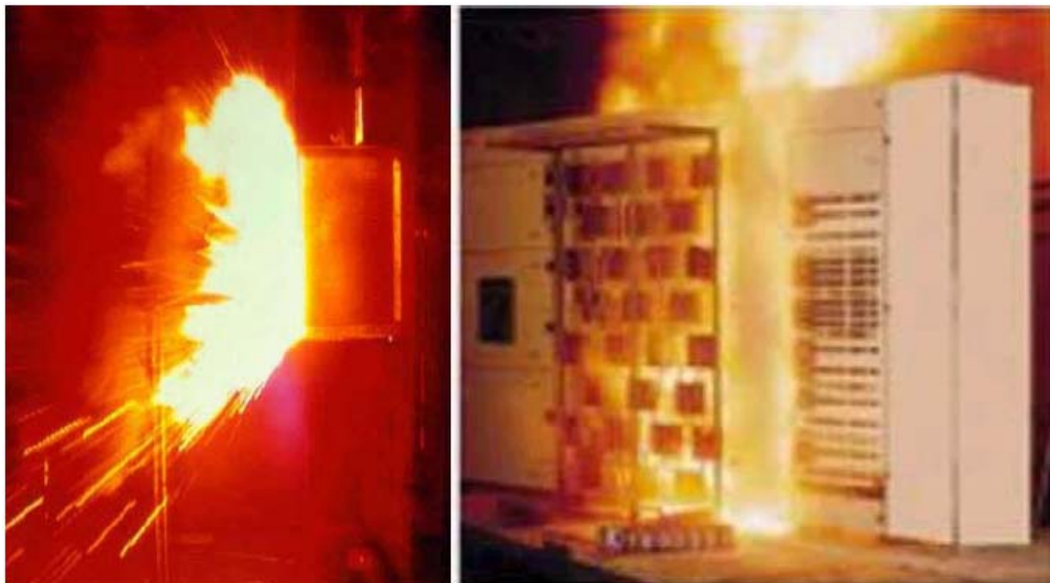
Figure 1.1: (a) Arc blast in box 2 ; (b) Arcing fault in electrical panel board
